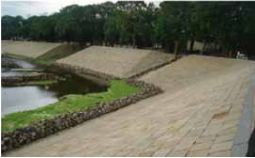
River bank protection
